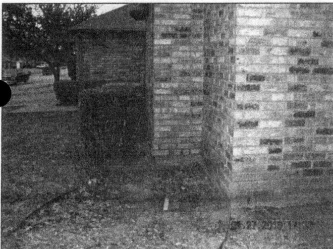
SOUTHEAST CORNER (LOWEST ADJACENT)
